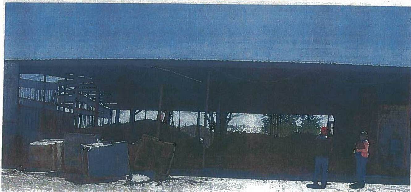
5-13-2010; 11:13 am Photograph # 1 Pecos Valley Meat, Roswell, NM Photographer: Teri Monaghan, NMED/SWB West side of covered canopy area containing offal and manure piles, facing east. Aurallie Ashley-Marx, NMED/SWB Chief and Eddle De Los Santos, brother of facility owner, assessing operation
